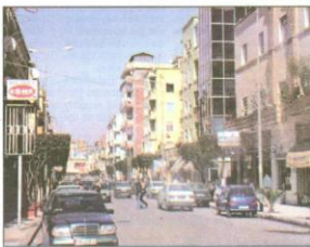
View of the Albanian central city of Durres where police codenamed operation "voltage" was conducted
